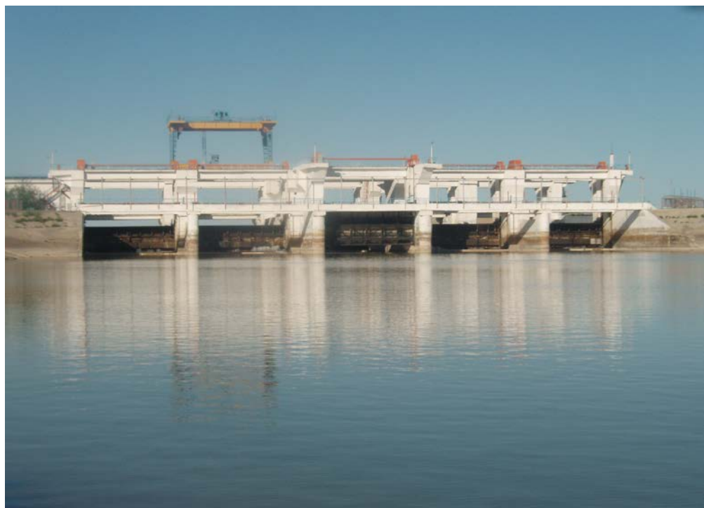
Fig.A7. Kazalinsk barrage.
