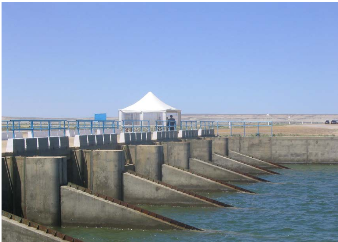
Fig.A3. Spillway at NAS dam.
