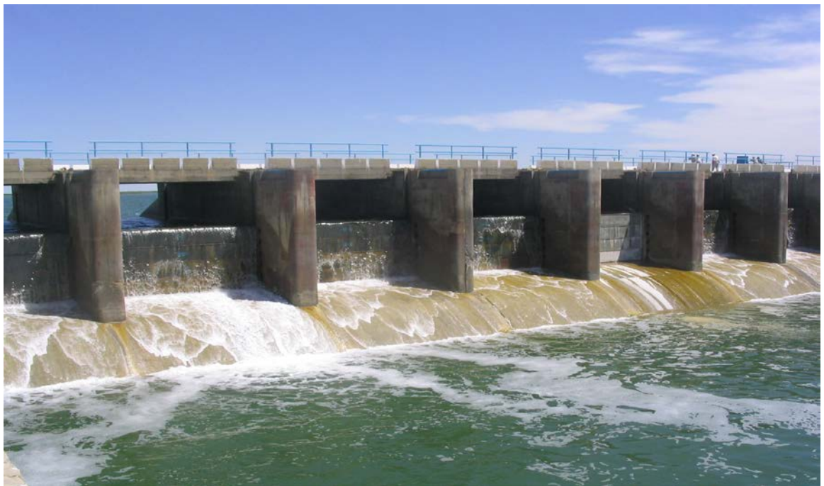
Fig.A2. Spillway at NAS dam.
