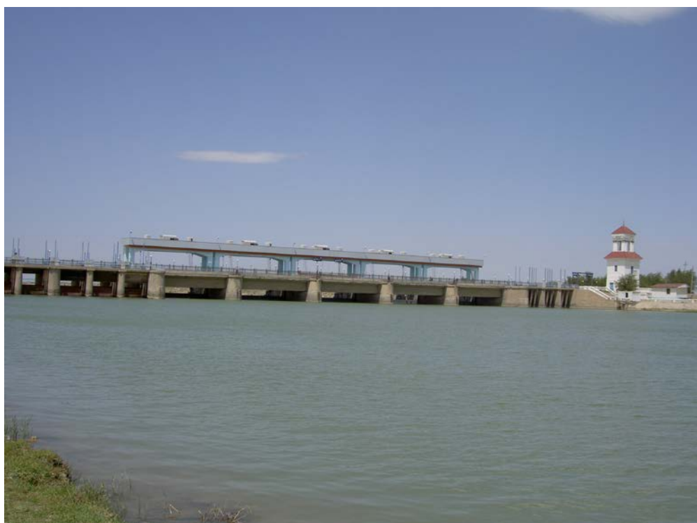
Fig. A8. Kzylorda barrage (upstream).
