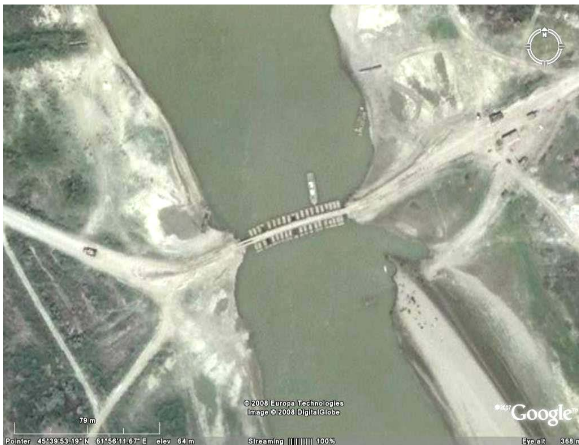
Fig. A11. Space image of existing pontoon ferry at Syrdarya river.
